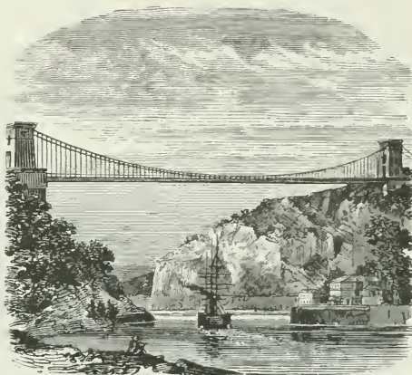
Fig. 66.—CLIFTON SUSPENSION BRIDGE.
